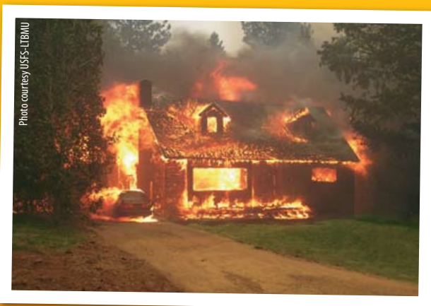
This house was ignited by burning embers landing on vulnerable spots. Notice the adjacent forest is not burning.
